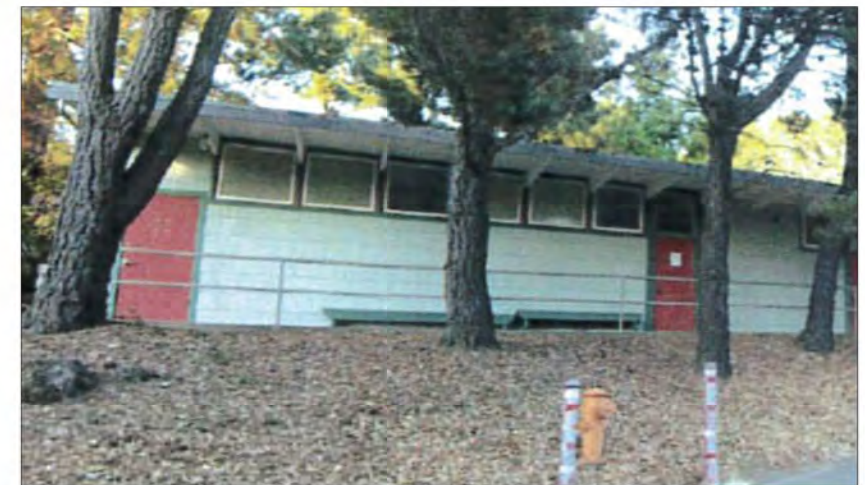
SITE 2: ANNEX BUILDING
