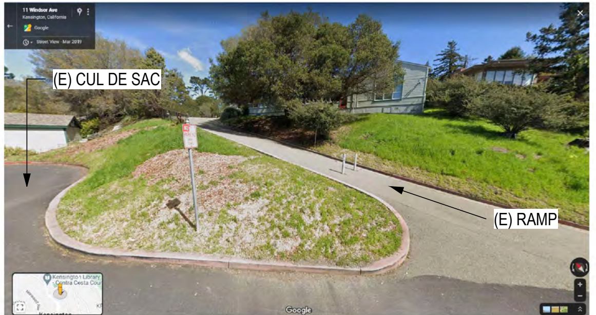
RAMP TO BULIDING E
