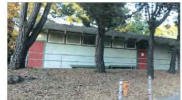
SITE 2: ANNEX BUILDING
