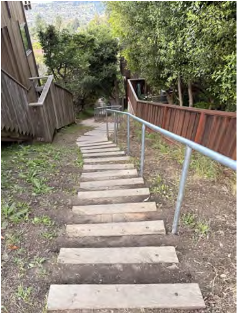
Beloit Lower - After with Handrail
