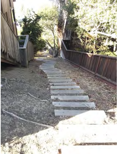
Beloit Lower - Before Handrail
