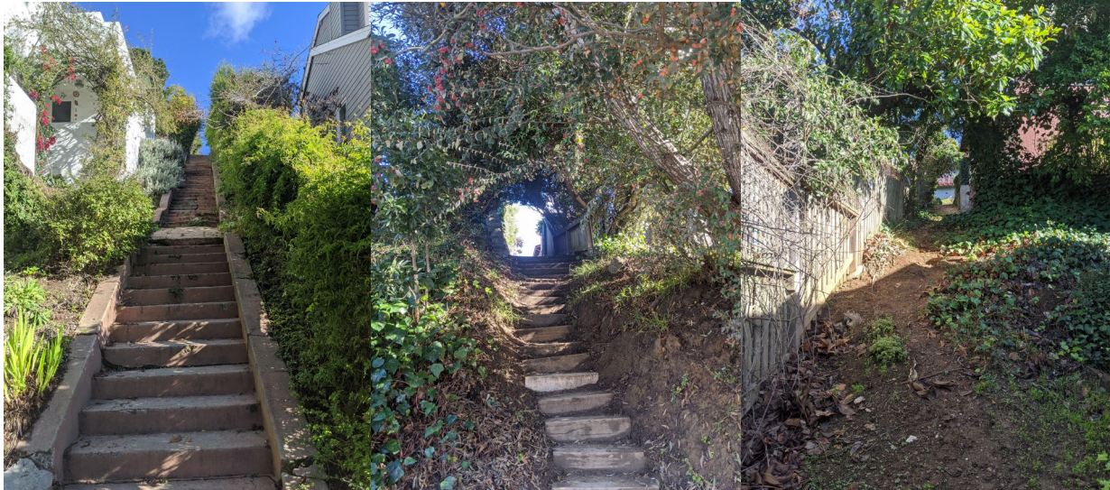
Figure 26: A range of path conditions in the northeastern quadrant, ranging from concrete surface to narrow, wooden stairs to an unmarked dirt trail. From left to right are Public Path #6 east of Arlington Avenue, the same path east of York Avenue with low overhanging foliage, and the Westminster path between Kenyon Ave. and Highland Blvd. All photographs were taken looking east.
