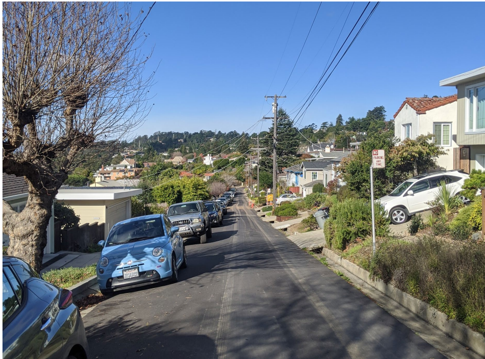
Figure 9: Cambridge Avenue, looking north from Beloit Avenue, showing a ~20' right-of-way narrowed to a maximum width of 18' by deep gutters (note non-navigable driveway crossings) and further narrowed to a minimum of 11' by parked vehicles.
