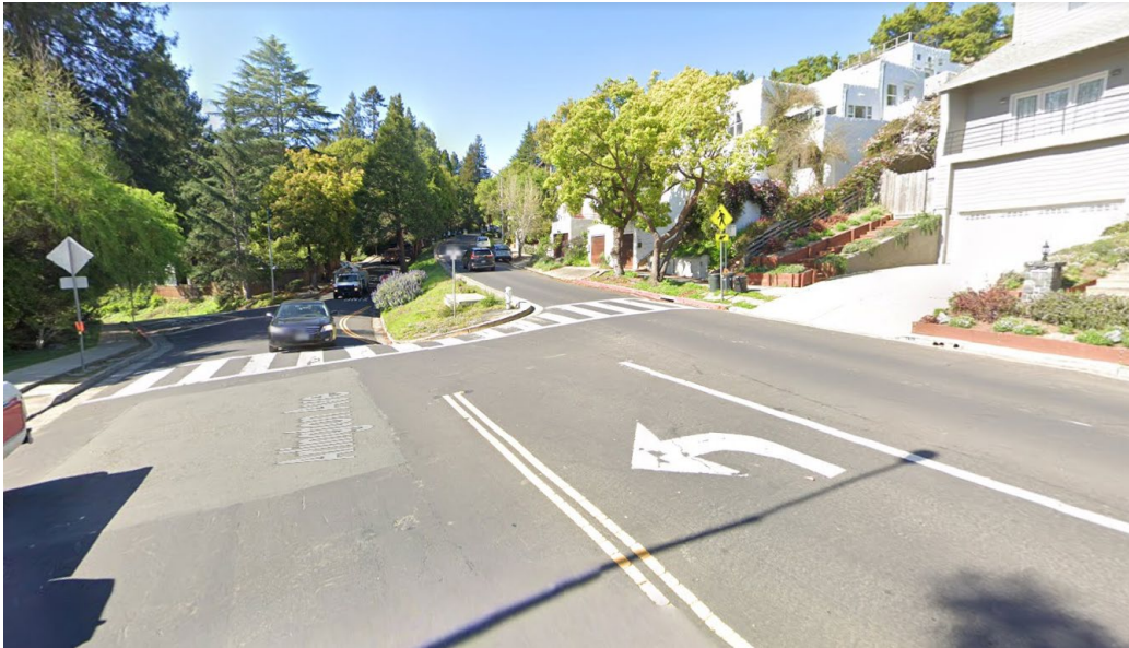
Figure 25: Another unconventional intersection is that of Arlington Avenue and Sunset Drive (shown here in Google StreetView). In this case, vehicles traveling from northbound Arlington Avenue to Sunset Drive must negotiate the turn lane here and then drive up a short segment of the southbound half of Arlington Avenue to then make another left on Sunset Drive (which branches to the left behind the car seen in the photo). Vehicles have also been observed using the median gap to exit Sunset Drive and make an immediate U-turn to proceed north on Arlington Avenue.
