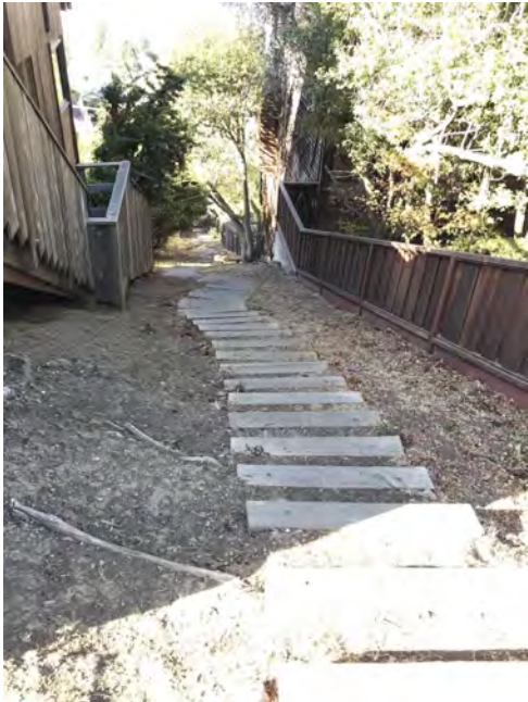
Beloit Lower - Before Handrail
