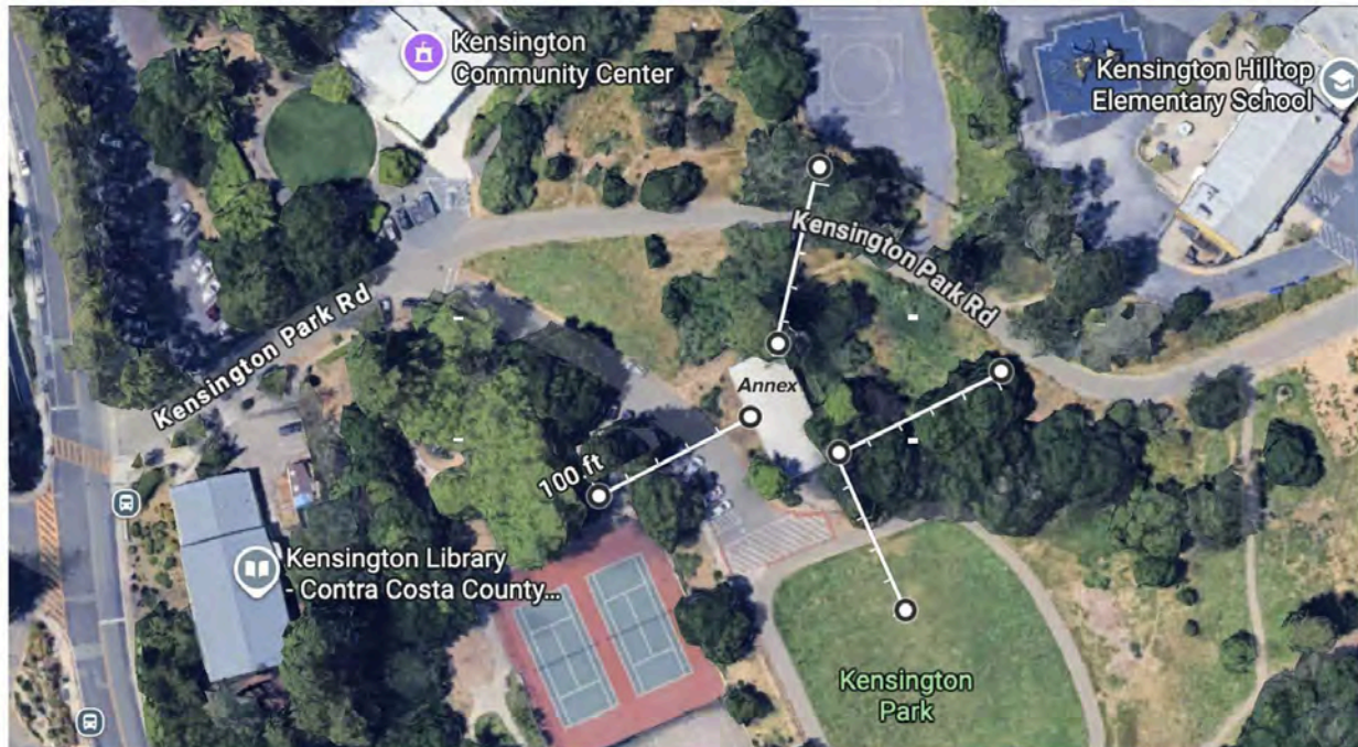
Photo: Aerial view of Annex building with 100' defensible space zone marked in white. Note the parking lot, tennis courts and picnic area to its west. Kensington Park Road walking path is upslope, winding around the building. The foot trail just north of the building cuts through the vegetation to the picnic area.
