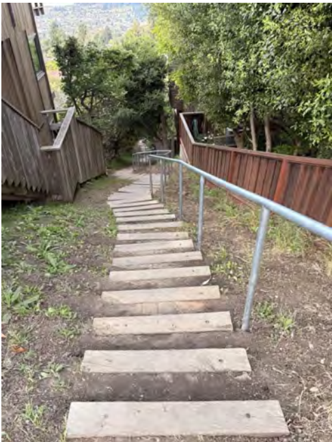
Beloit Lower - After with Handrail
